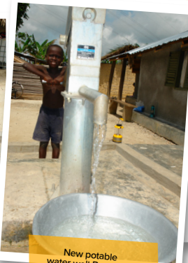
New potable water well Bompieso
